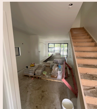
Group C internal painting underway on the ground floor.
