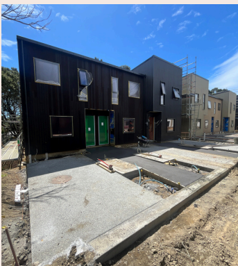
Group A driveways and pathways poured, and cladding freshly stained.
