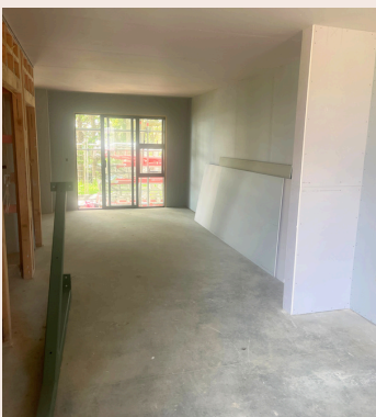
Group D Gib installation downstairs
