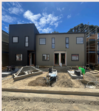
Group C cladding detailing
