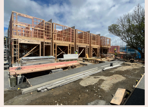
Group F framing up and pathways poured. Trusses delivered 15/11.
