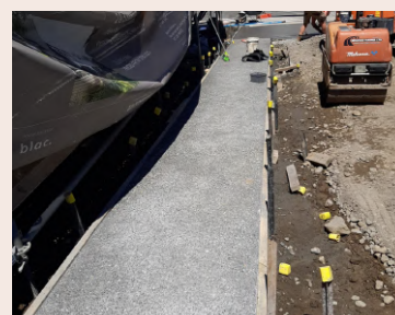
Pathway at main entrance, adjacent to Group G.
